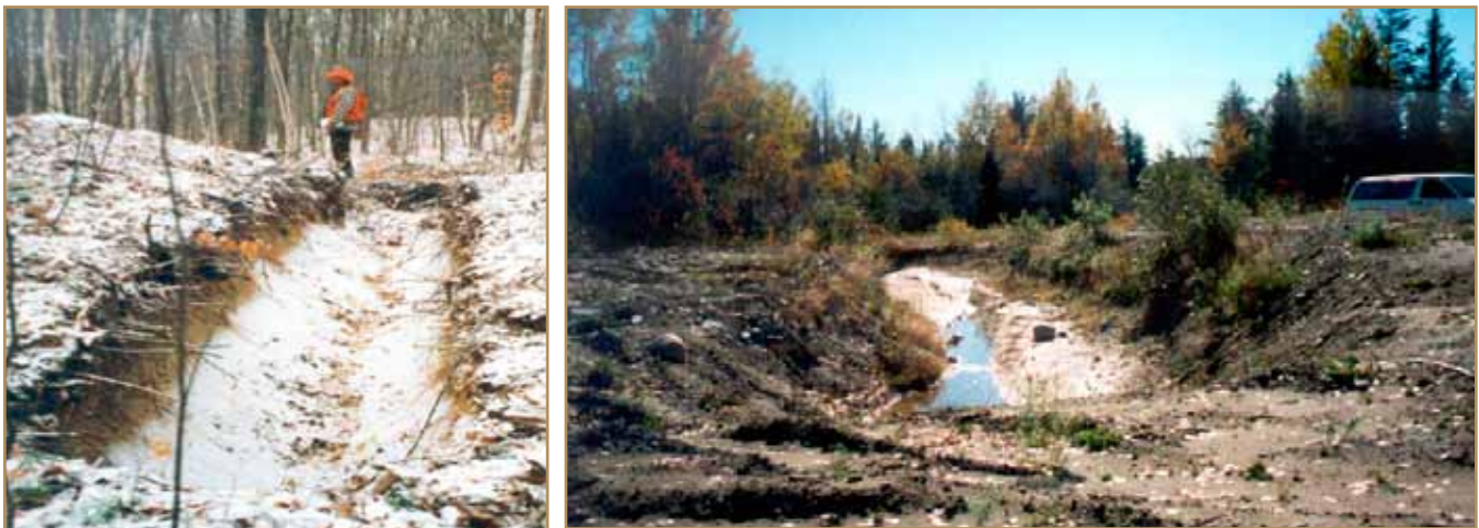
Figure 4: Examples of power stripping
