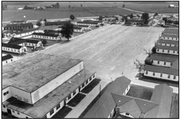
Camp Ipperwash's H-Hut barracks were home to over 1500 cadets every summer. Circa 1986
